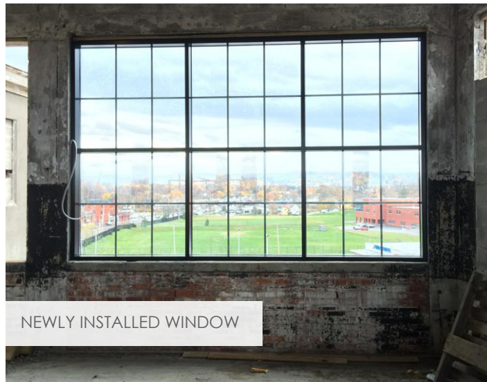
NEWLY INSTALLED WINDOW
